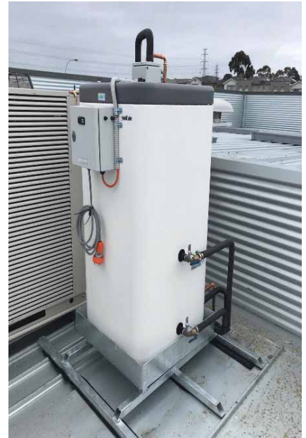
A large commercial restaurant is using an air-conditioner as an initial heat source for commercial hot water needs.
