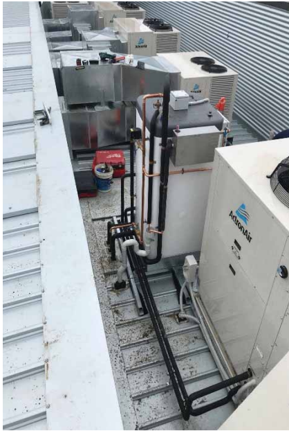
A large commercial restaurant is using an air-conditioner as an initial heat source for commercial hot water needs.
