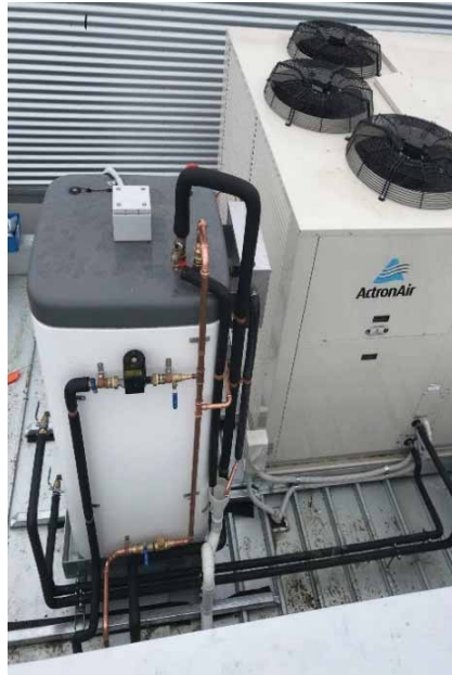
A large commercial restaurant is using an air-conditioner as an initial heat source for commercial hot water needs.
