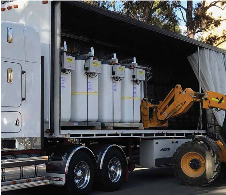
Plug and play packaged systems can be delivered to projects for final water and power supply connections which greatly saves in labour and material costs onsite.
