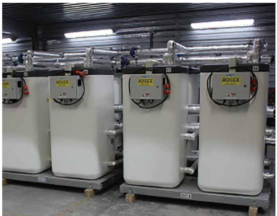
Rotex thermal storage can be used for many heating and cooling applications.
